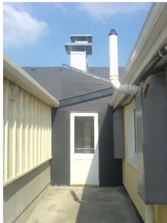
Example of Ducting from a Magnacooler
